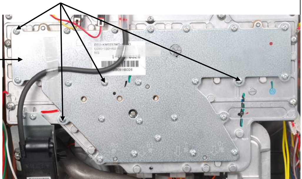
Cover Plate Retaining Screws
