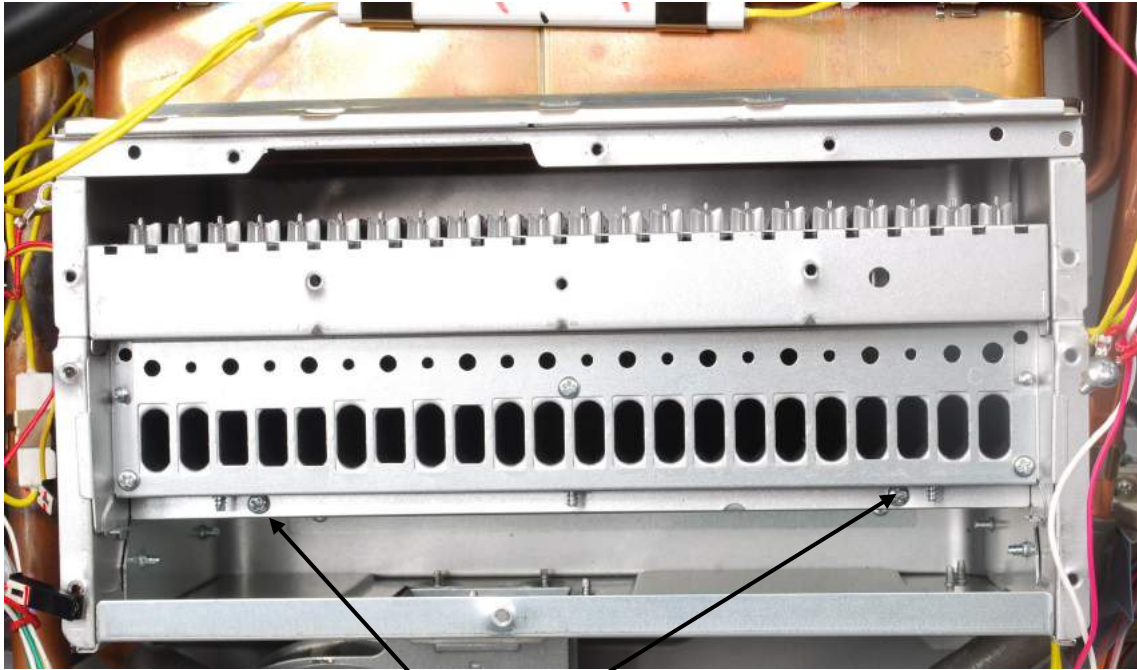
Burner Box Screws
